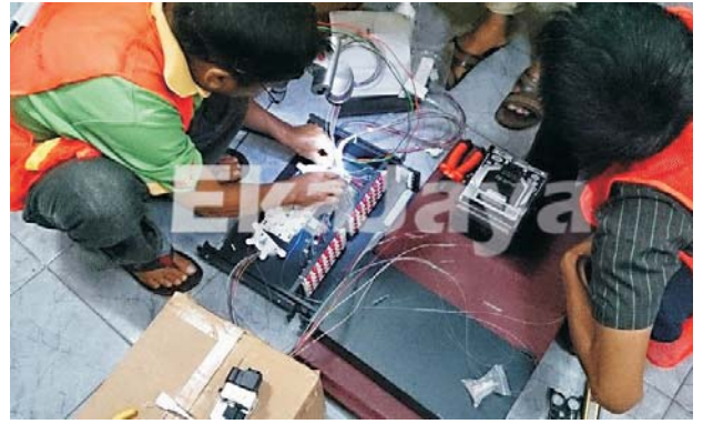
Terminasi FO metode Fusion Splicing
